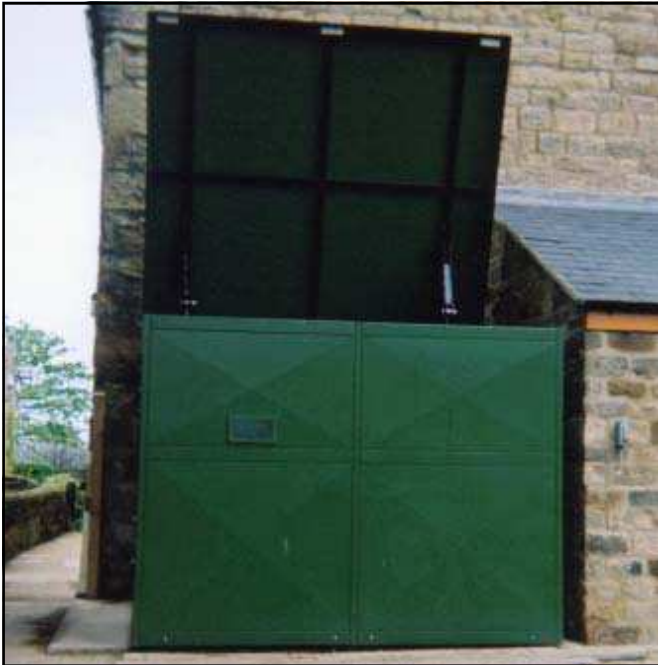
Above; Hydraulic hopper lid open for fuel loading. Below; The purpose built boiler house and Econergy designed steel hopper
