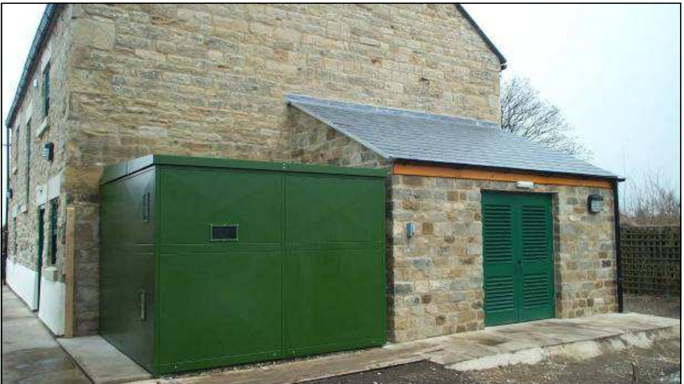
Above; Hydraulic hopper lid open for fuel loading. Below; The purpose built boiler house and Econergy designed steel hopper
